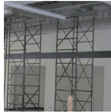
Masonry wall prior to demolition.
