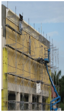
Renovation of a commercial plaza located in Venice, FL.
