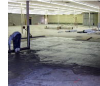
Beginning phase of retail remodeling.
