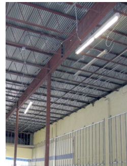
New structural support system in place.
